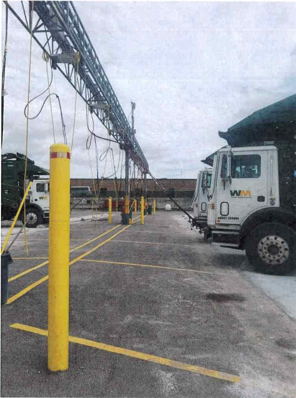
Figure 4: Typical CNG Fleet Vehicle Fueling Connection
